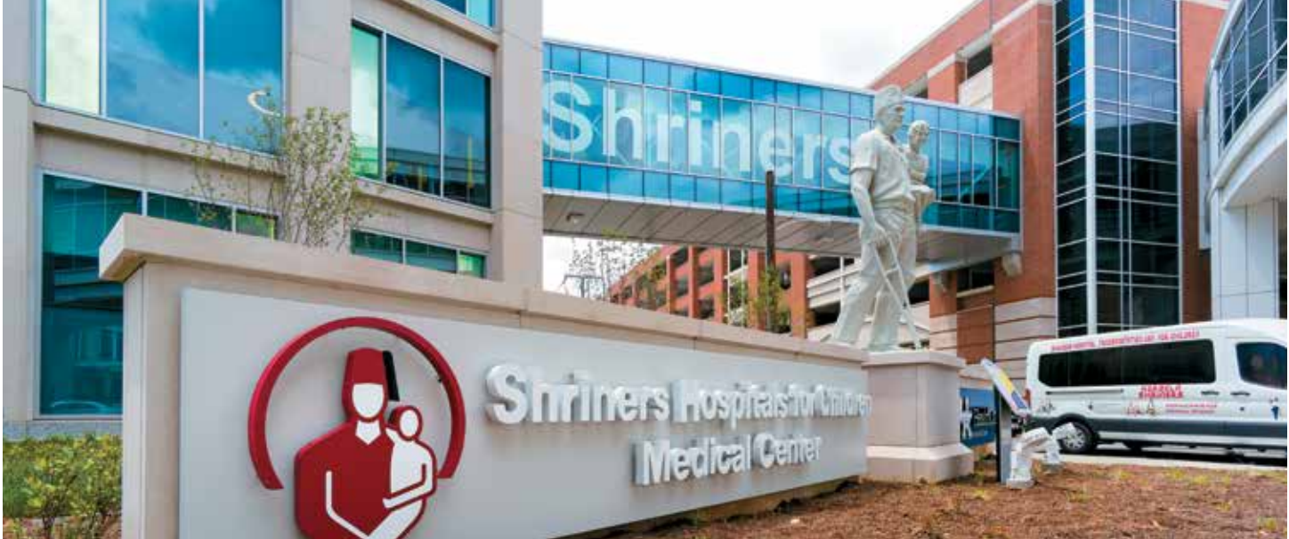
Pedestrian bridges connecting Shriners Medical Center with the Children’s Hospital underscore a longtime collaboration.
